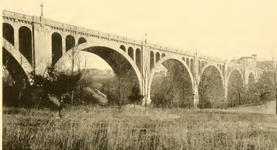
Connecticut Avenue Viaduct over Rock Creek Drive, just East of Massachusetts Avenue Park
