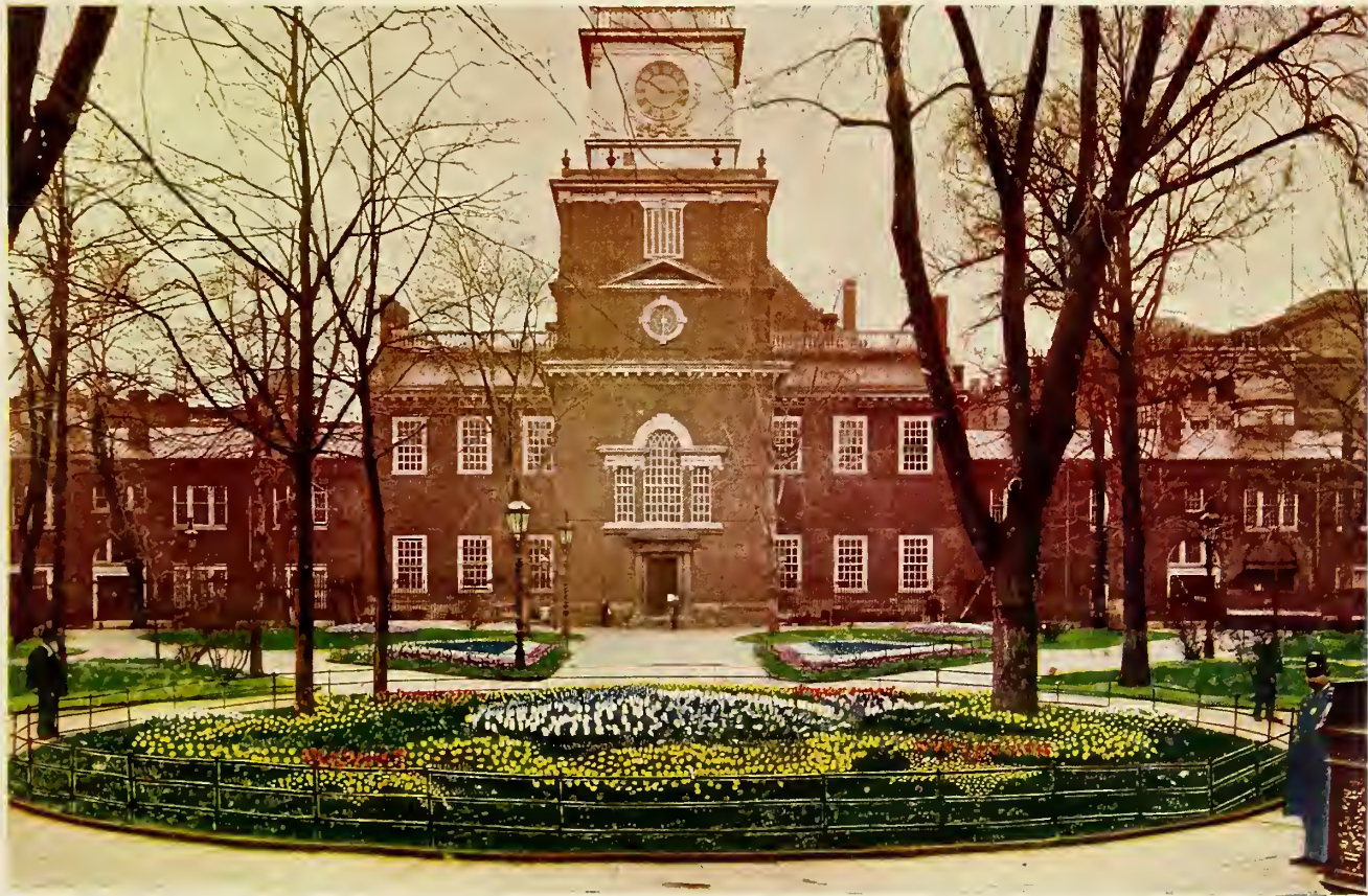
View of Independence Square, taken April 25, 1897, showing part of 65,000 Hyacinths, Tulips, Daffodils and Crocus, planted under directions of City Forester JOHN C. LEWIS, who reported that every bulb bloomed and was true to name and color. All Bulbs supplied by us.
