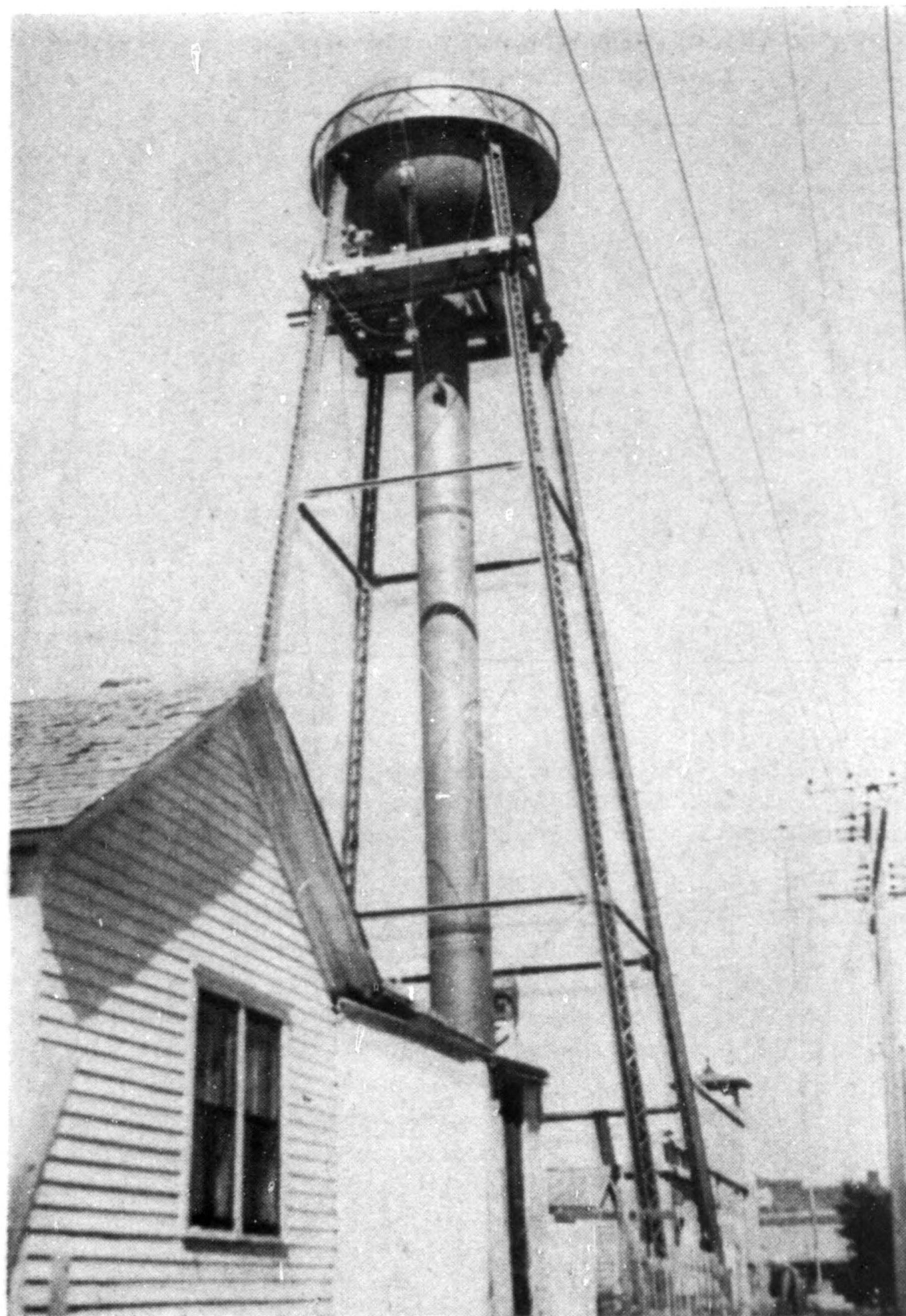
New water tower being erected at Wishek.
