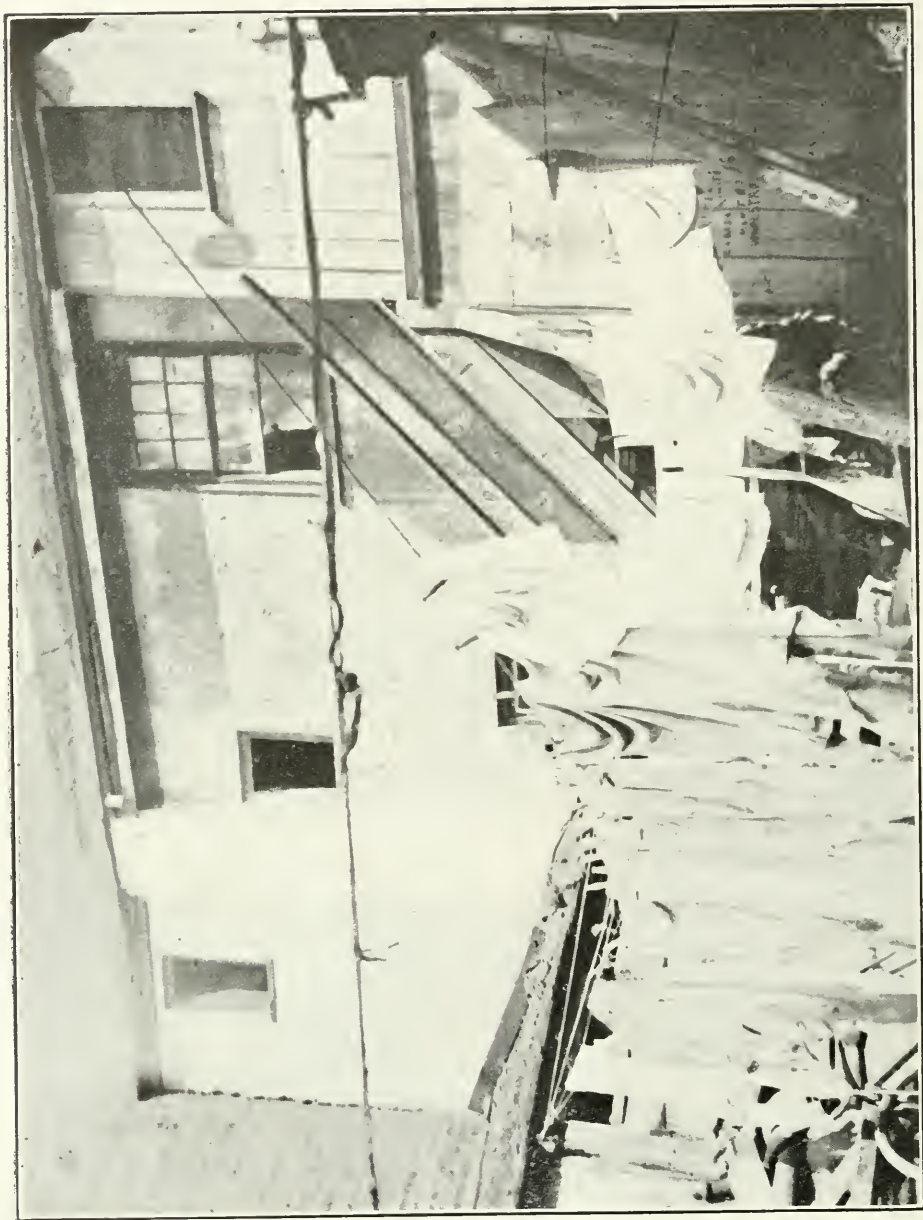
Rear view of a two-roomed dwelling over a store. This stair is the only means of access. — Burnett.
