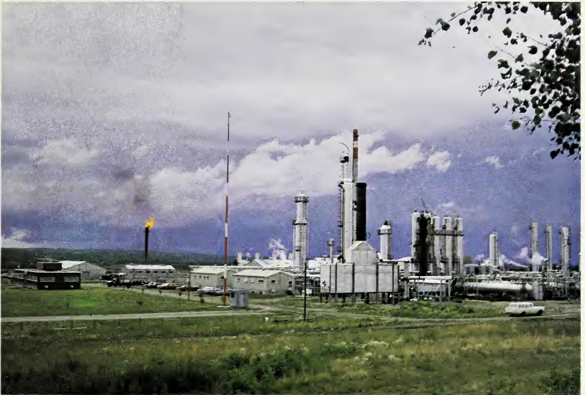
New processing plants, such as this one at Rimbey, have contributed greatly to the dramatic increase in the production, sale and distribution of natural gas over the past few years.
