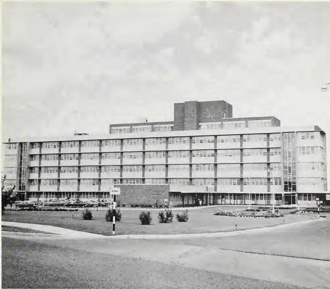
The Medicine Hat Municipal Hospital, typical of the modern, efficient health care facilities available to all Albertans.
