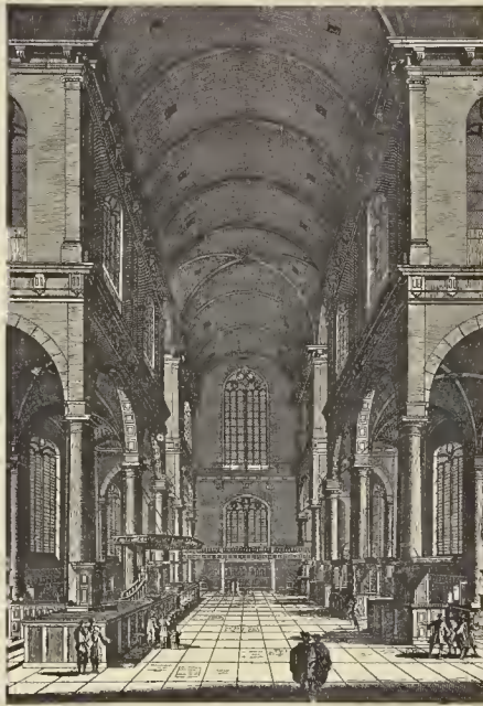
INTERIOR OF THE WESTERKERK. (Facsimile of a contemporary Print.)
