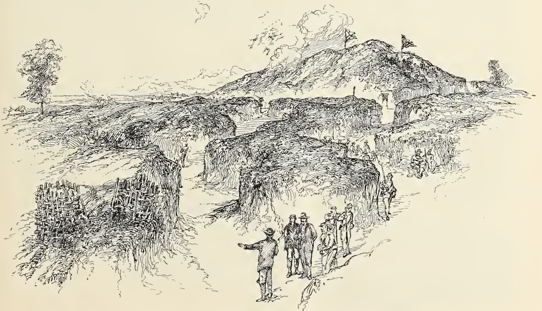
VIEW OF VICKSBURG DURING THE SIEGE, FROM THE FEDERAL TRENCHES.
