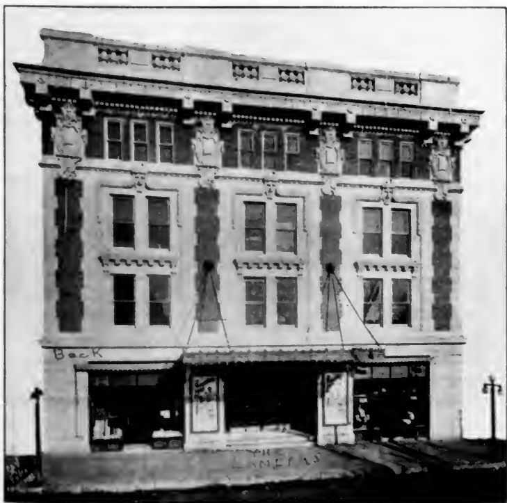
The Landers Theatre, of Springfield, Missouri, is one of the most beautiful structures in Southwest Missouri. The cost of the building was $201,000. The seating capacity is 1,400. It has a stage front of 55 feet. Mr. George Olenhoff is the manager and is booking with K. & E. Circuit.
