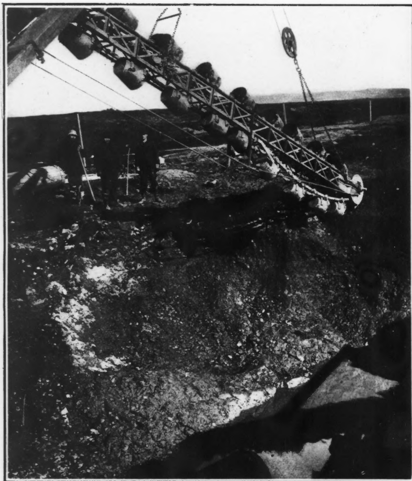
LAYING BEDROCK DRAIN FROM SEA TO THIRD BEACH LINE, BOURBON CREEK
