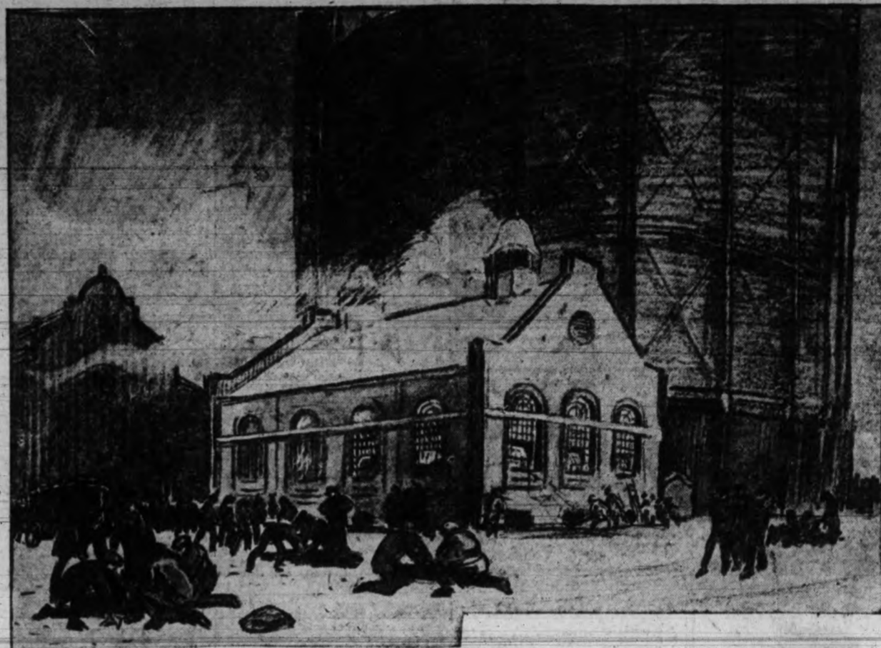
Ten men were killed, and nearly a score of others temporarily overcome, by escaping gas at the plant of the Consumers' Gas Company, Toronto, on February 8. Above is shown the outside of the building, with relief parties working over the bodies of the victims as they were carried out.
