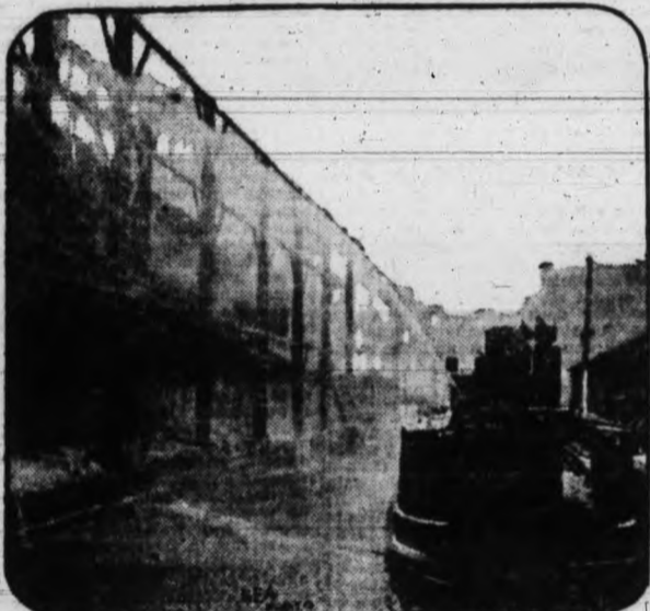
Undismayed by wintry blasts and difficulties of location, Erie, Pa., firemen converted a commercial tug into a fire-fighter when a $100,000 blaze destroyed the Keystone Fish Company buildings there recently. Hose was carried across channels on rowboats.
