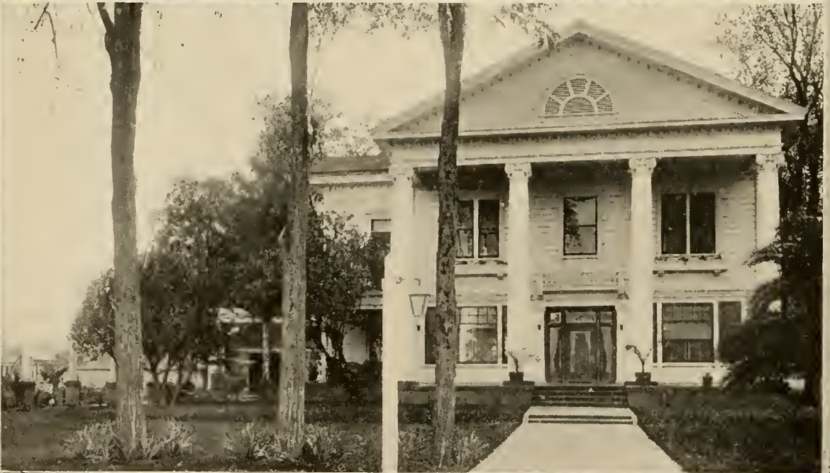
EVIDENCES OF PROSPERITY ON THE FARM. EVERYWHERE IN YOLO COUNTY IS FOUND THE COMFORTABLE HOSPITABLE HOME
