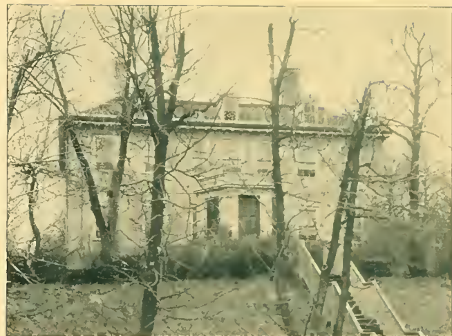
THE SCHUYLER MANSION—ERECTED IN 1760-61
