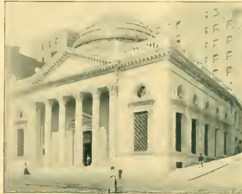
ALBANY SAVINGS BANK
