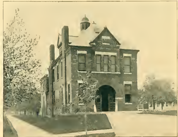
ALBANY FIRE DEPARTMENT—STEAMER HOUSE No. 10
