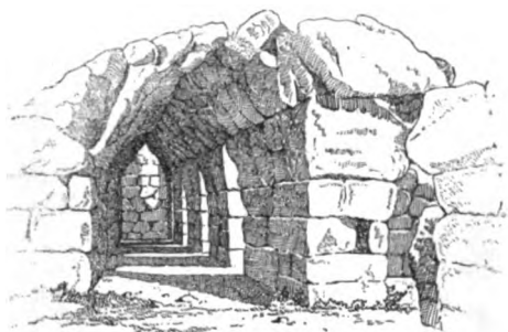
FIG. 74. GALLERY IN THE SOUTH WALL AT TIRYNS
