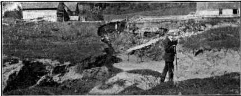
FIG. 1.—Gully encroaching on farmer's premises which, unless controlled, will undermine the buildings. Near Alma, Wis.
