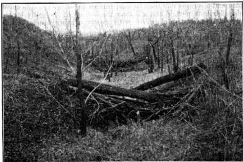
FIG. 11.—Gully formerly deep with steep banks reclaimed by locust trees and brush dams. Near Martin, Tenn.
