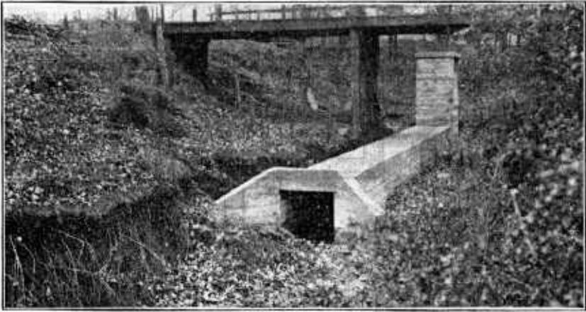
Fig. 27.—Highway bridge to be replaced by an earth embankment and a combined culvert and concrete drop inlet. Near Winterset, Iowa
