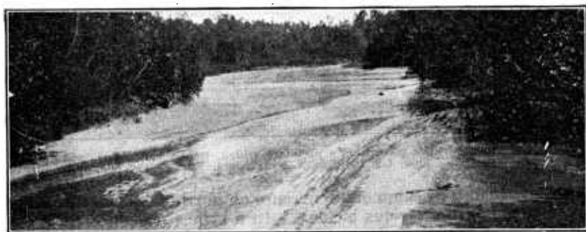
FIG. 3.—Channel nearly filled with sand washed from adjoining hills, requiring dredging at great expense to provide drainage for the bottom lands. Gwinnett County, Ga.
