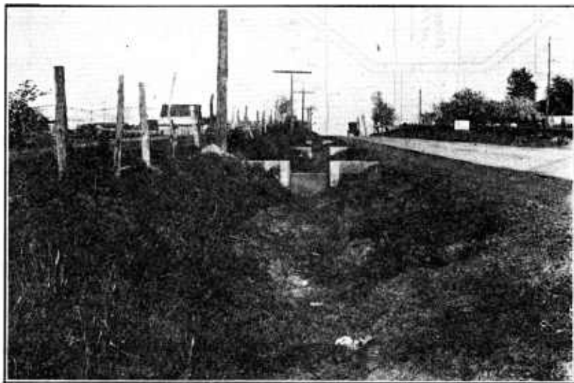
FIG. 22.—Series of reinforced concrete dams used to check erosion
