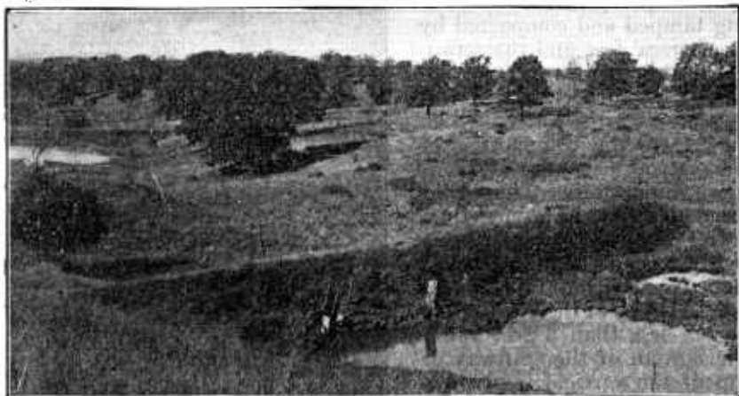
FIG. 26.—Two large earth soil-saving dams in one draw where formerly a gully existed. Near Warrensburg, Mo.
