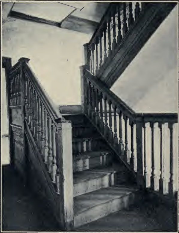
Illus. 421.—Stairs at "Graeme Park," Horsham.
