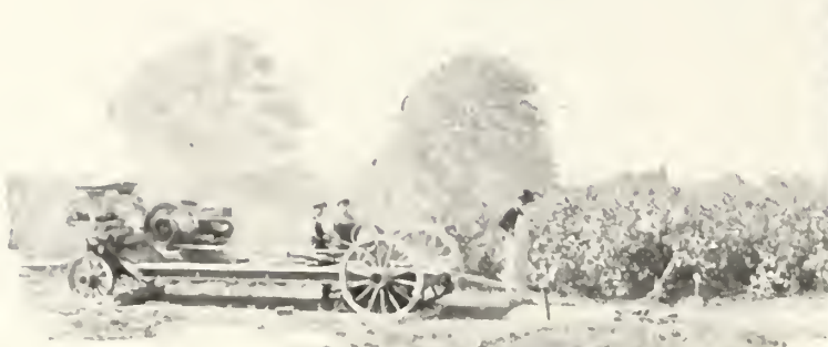
Gas engine and windlass to pull L-blade root pruner, invented by Valentine Wickey, Superintendent Tree Moving Department, Hicks Nurseries. Root pruner is pulled by a wire cable.
