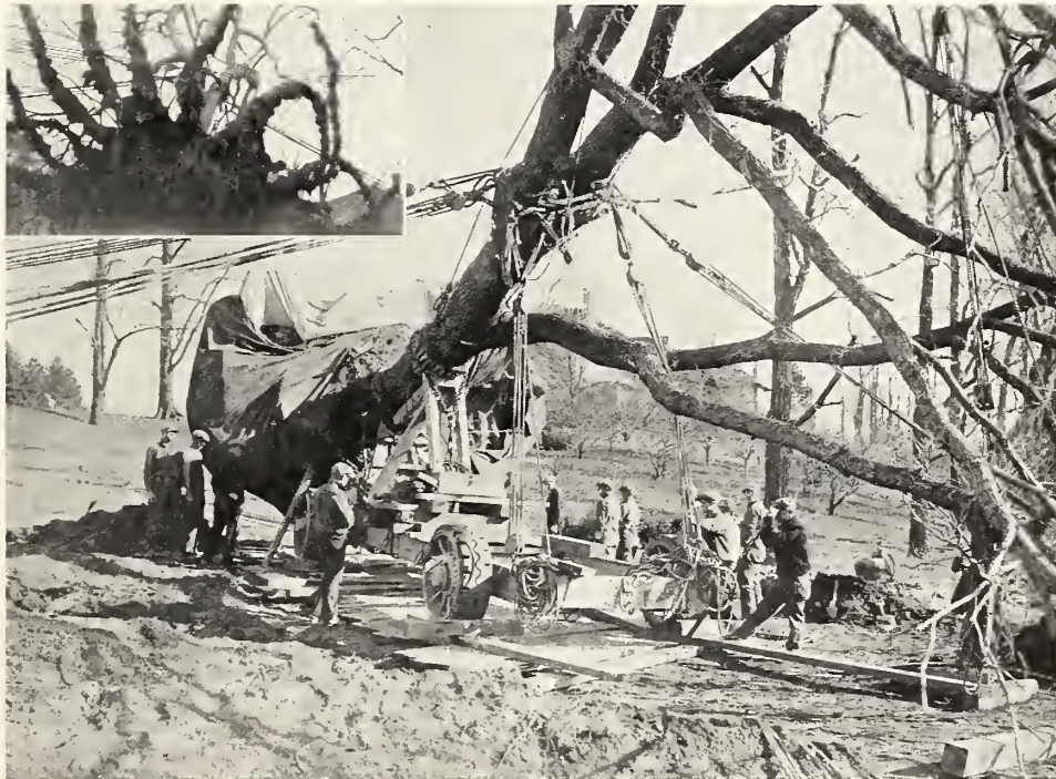
Large elm being moved for Mr. Howard W. Maxwell, Glen Cove, L. I. Ferruccio Vitale, Landscape Architect. The tree is 29 inches in diameter, 70 feet high and 80 feet spread, yet our men and apparatus handle it with ease. The insert shows how all the roots are saved by carefully picking out, tying in bundles and wrapping in straw. The bundles of roots are then wrapped around the center ball of earth and covered with canvas to prevent drying out.
