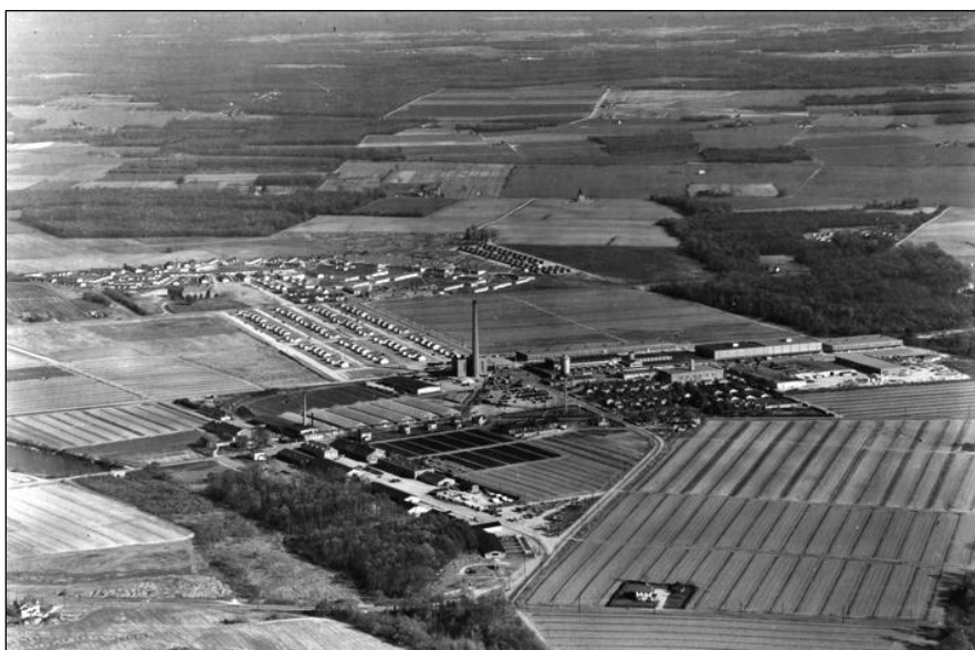
Aerial photo showing the Seabrook Farms plant and factory in about 1949. Photo courtesy of Seabrook Museum and Cultural Center
