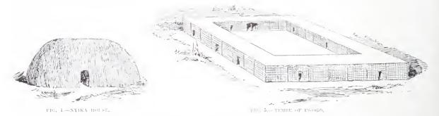
much as 15 feet long. Sometimes they are divided into two or more compartments. The framework is made of slender poles bound together with withes and forest vines, and all is covered with a thick thatch of grass which extends to the ground.
