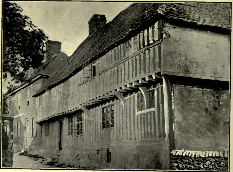
OLD HOUSE, HOLLINGBOURNE
