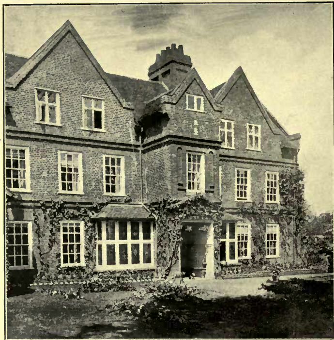
CEDAR HOUSE, HILLINGDON
