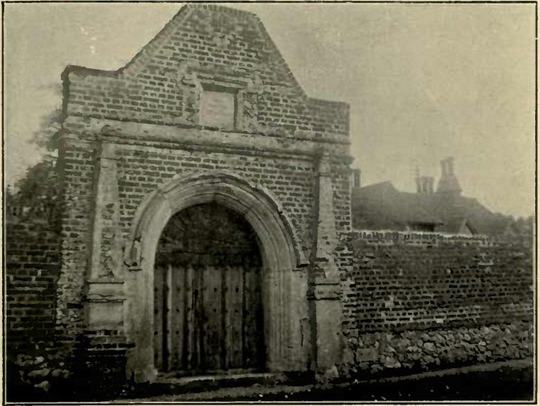
GATEWAY, DAVINGTON COURT
