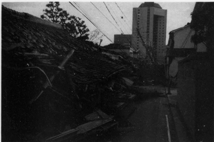
Heavy tile roofs on old wooden houses figured in most of the cases of collapsed buildings.
