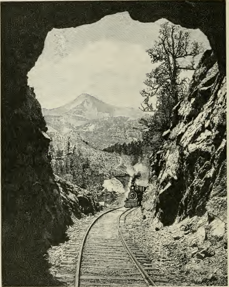
Portal of a Finished Tunnel ; showing Cameron's Cone, Colorado.
