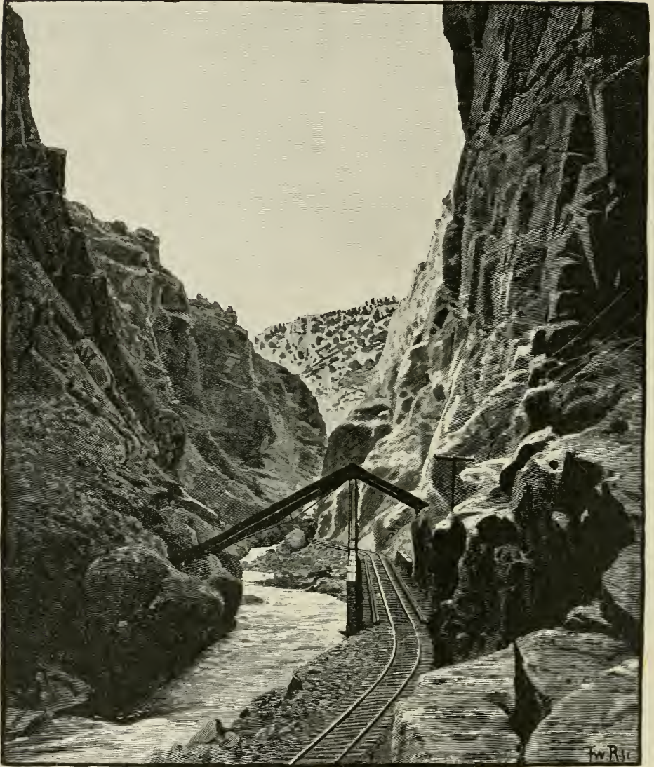
Royal Gorge Hanging Bridge, Denver and Rio Grande, Colorado.
