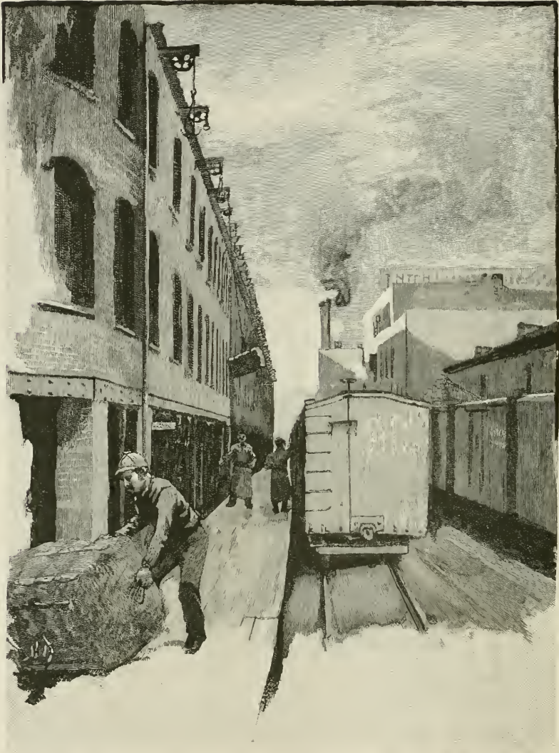
Hay Storage Warehouses, New York Central & Hudson River Railroad, West Thirty-third Street, New York.
