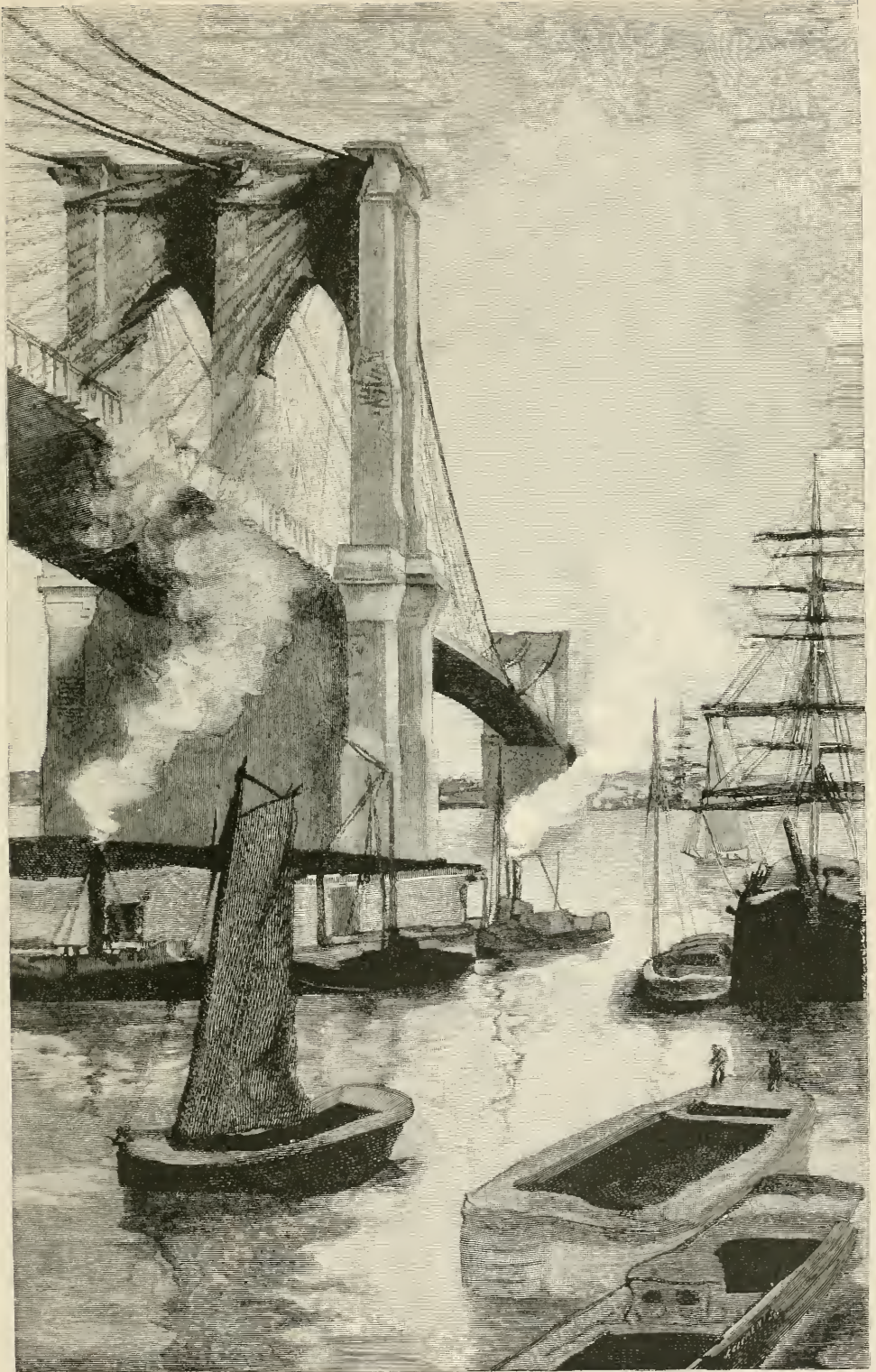
Below the Brooklyn Bridge. From a painting by J. H. Twachtman.
