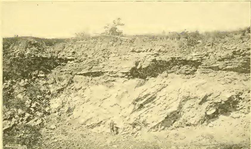
FIGURE 1. Exposure of LeClaire limestone at the Sugar creek lime quarries, Cedar county, Iowa. The limestone is obliquely bedded in the lower part of the section and horizontally bedded above. The same fauna occurs in both sets of beds. Oblique beds dip southeast.
