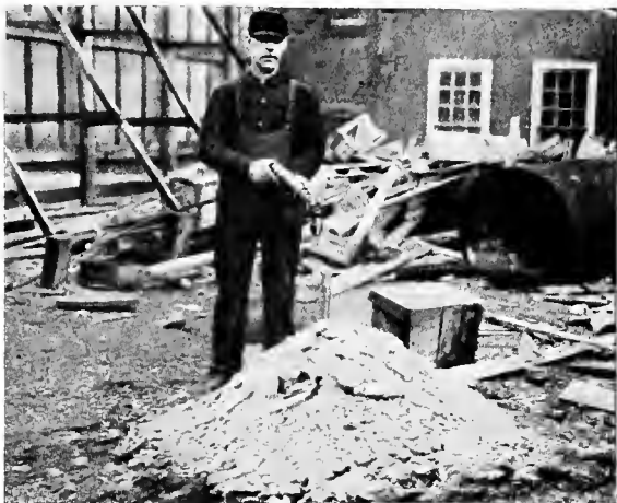
FIG. 19.—Scale removed from a boiler. (From Fower , Dec. 22, 1914.)
