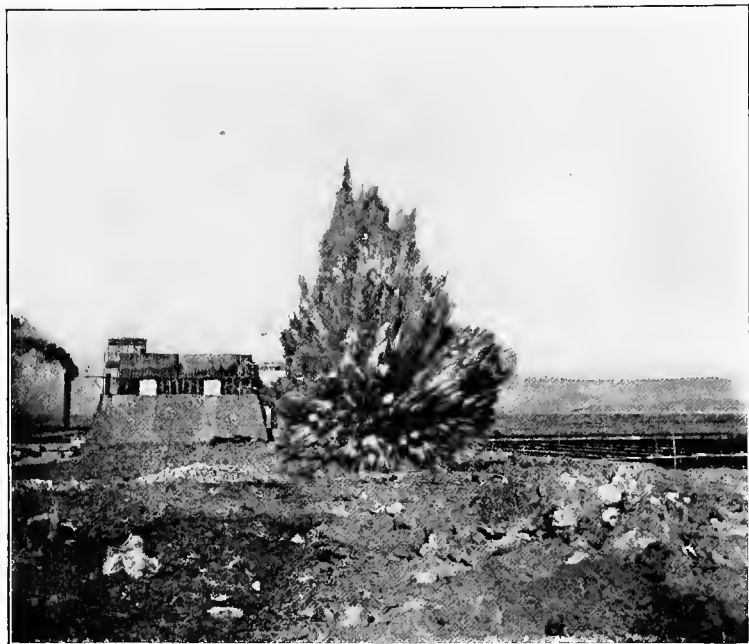
FIG. 45.*—Blasting a test hole in caliche to obtain nitrate of soda.
