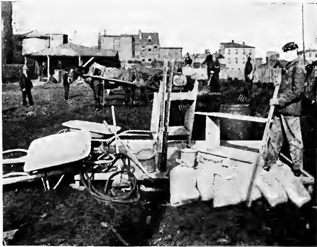
FIG. 79.—Concrete board and tools for making concrete. (Farmers' Bulletin 461, U. S. Dept. Agr.)
