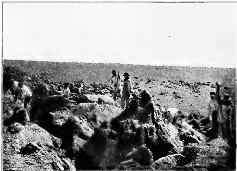
FIG. 46.—Opening up a trench after blasting; extraction of caliche by piece work.
