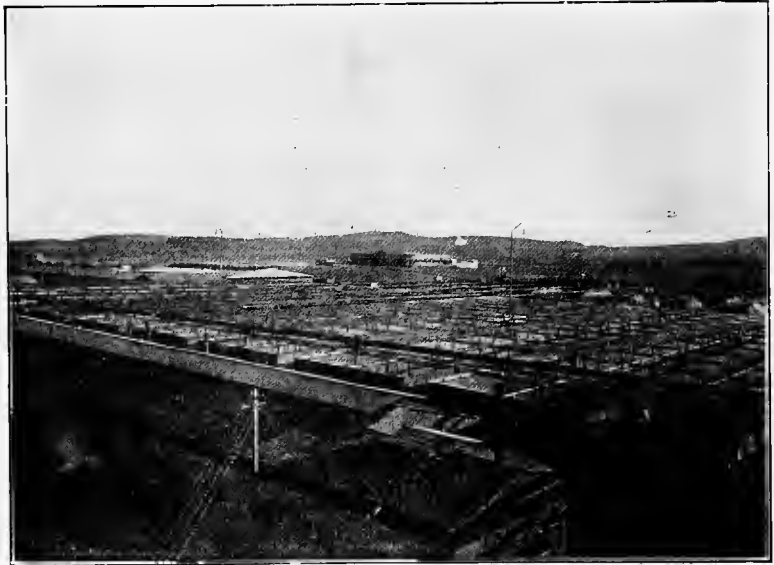
FIG. 48.—General view of crystallizing pans for obtaining nitrate of soda. Each pan has about 500 cu. ft. capacity and 225 sq. ft. cooling surface.
