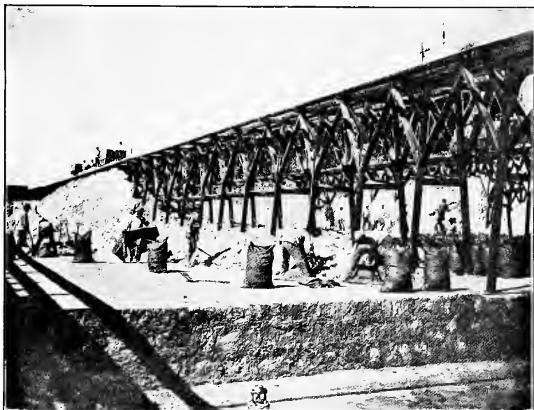
FIG. 50.—Drying floors and bagging of nitrate of soda.
