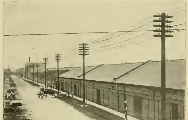
FIG. 2.—500,000 CIRCULAR MIL FEED LINE.
