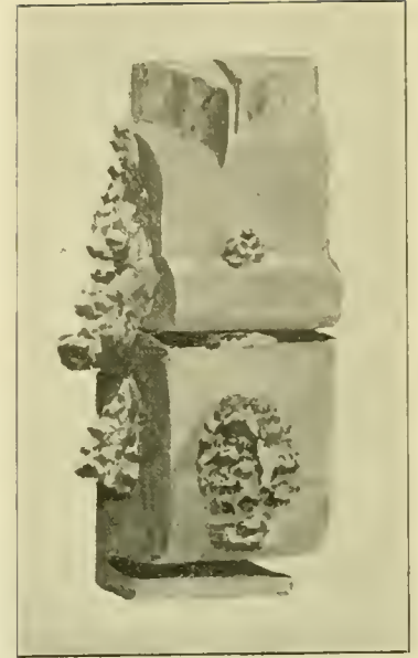
LUG KNOCKED OFF DEFECTIVE ELECTRIC WELD.
