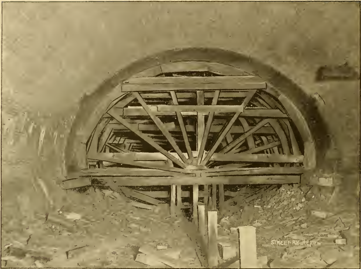
INTERIOR OF TUNNEL DURING CONSTRUCTION, SHOWING METHOD OF BRACING.
