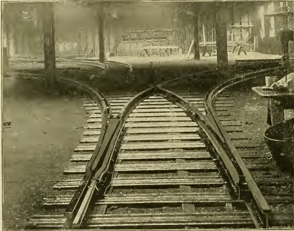
PAIGE IRON WORKS—SINGLE TRACK T RAIL Y CURVE BUILT OF ILLINOIS STEEL COMPANY'S SHANGHAI T RAIL. SET ON DANIELS STEEL TIES.
