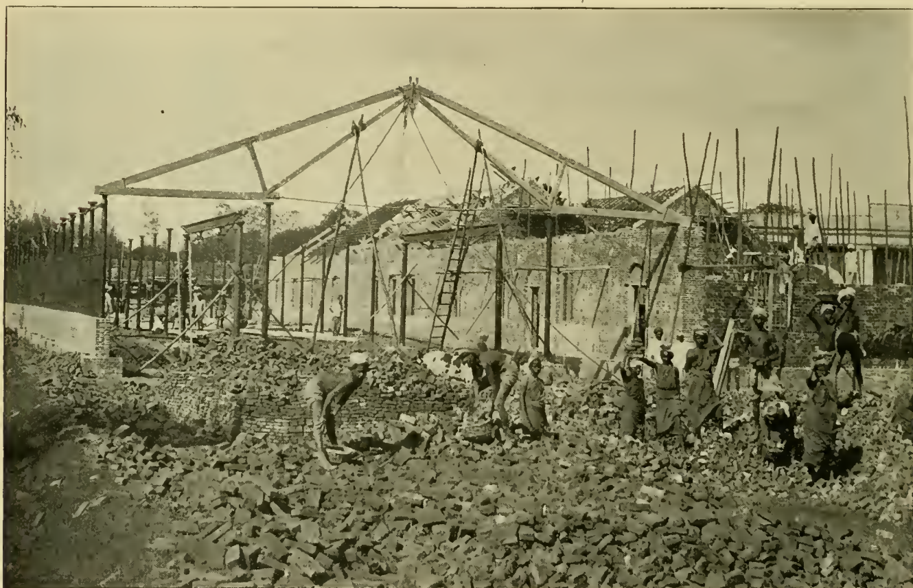
MADRAS ELECTRIC TRAMWAY—WORK COMMENCED ON CENTRAL POWER STATION.
