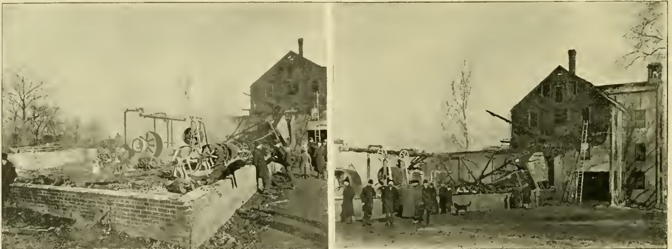
RUINS OF THE ATTEBORO, MASS., POWER PLANT.
