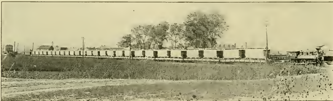
"The first section carried twenty-seven cable cars"
