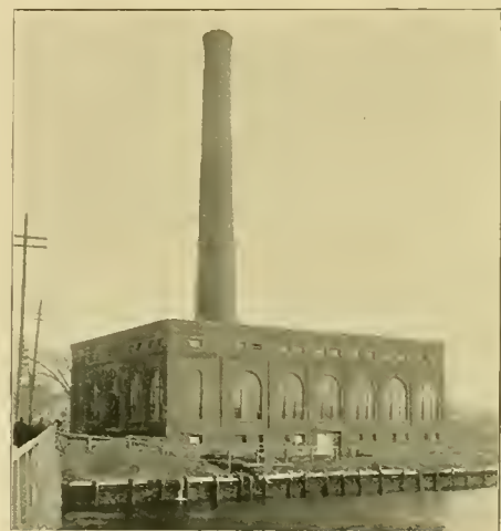
EXTERIOR OF POWER HOUSE.
