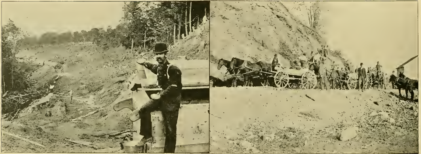
CONSTRUCTING THE LINE.
