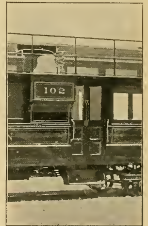
PULLMAN CENTER ENTRANCE.
