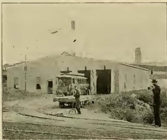
EAST SIDE POWER-HOUSE—ATLANTA TRACTION.
