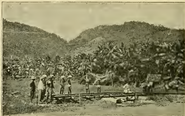
CONSTRUCTING THE LINE.
