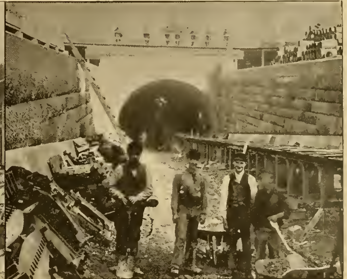
WEST APPROACH OF TUNNEL SIXTY DAYS LATER.
