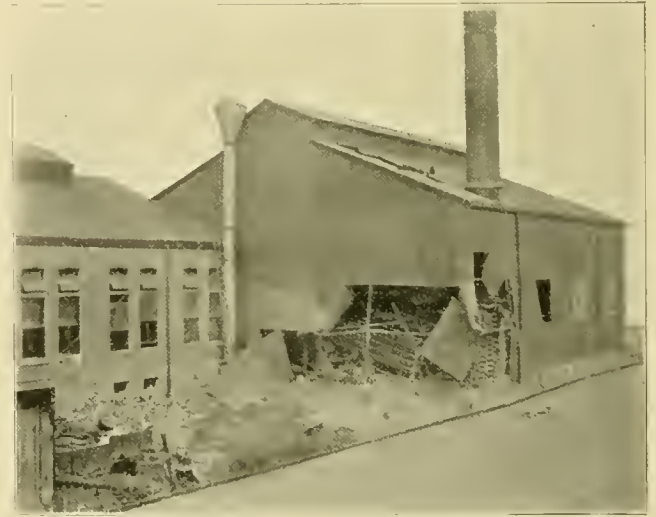
NATURAL GAS EXPLOSION, INDIANAPOLIS.
