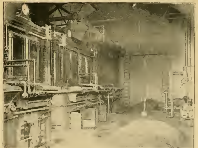
BOILER ROOM, NEWPORT POWER STATION.
