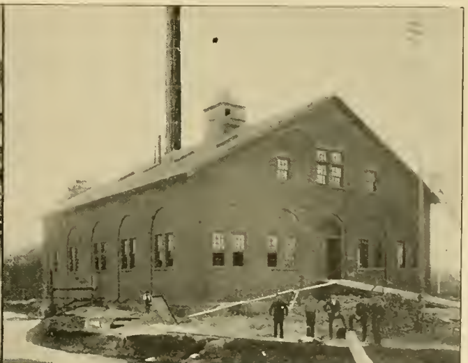
POWER HOUSE AT JOHNSTOWN.
