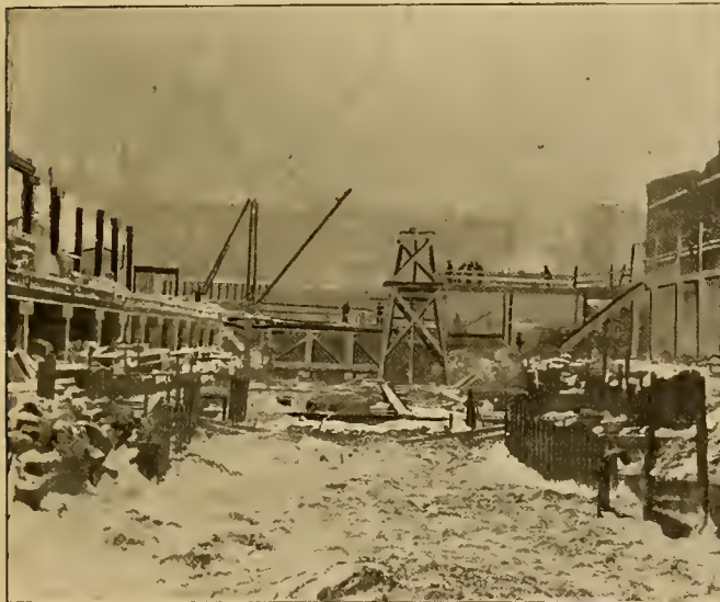
WEST APPROACH OF TUNNEL ON JANUARY 15, 1894.
