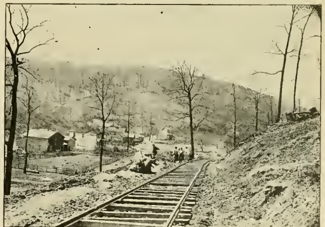
CONSTRUCTING THE LINE.
