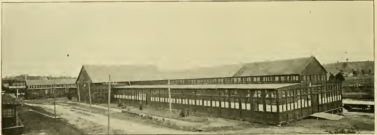
MACHINERY HALL, WHERE CONVENTION WILL BE HELD.
