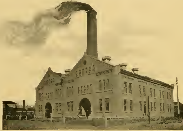
THE WHEELING POWER HOUSE.
