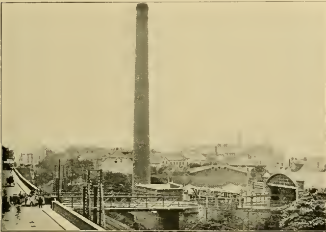
VIEW OF POWER HOUSE AND RAILROAD VIADUCT—BARMEN.
