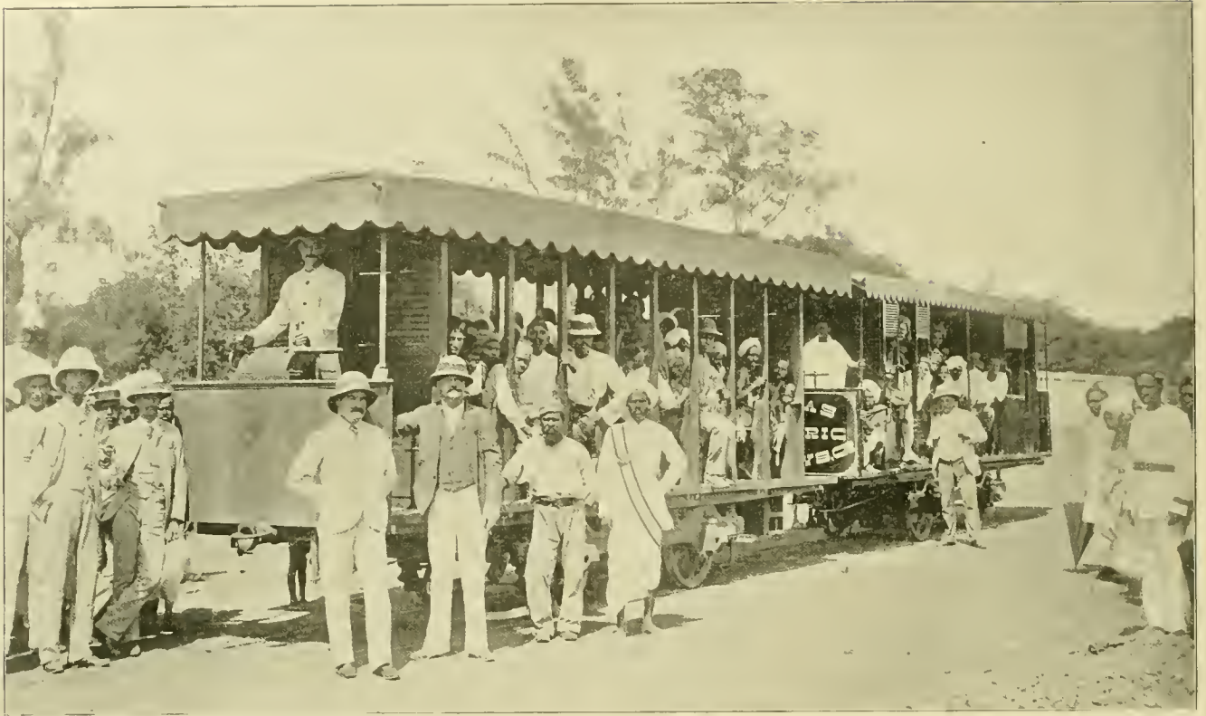
MOTOR CAR AND TRAILER OF AN ELECTRIC CONDUIT ROAD—MADRAS, INDIA.
