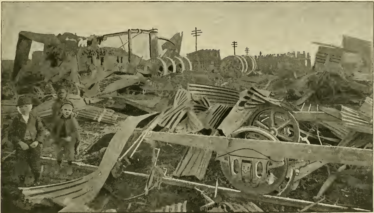
RUINS OF CAR HOUSE—SAVANNAH ELECTRIC RAILWAY.
