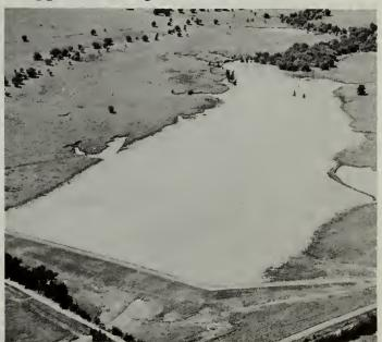
This floodwater retarding dam in Frog Creek Watershed, Coffey County, reached its flood storage capacity when 11 inches of rain fell in three days in June 1967. Benefits from the 11 dams in the watershed were estimated at \$132,000, while millions of dollars of damage occurred in unprotected watersheds in that period.
