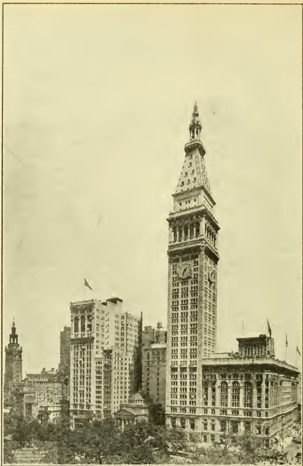
The Metropolitan Tower, Madison Square. Madison Square Garden on the left
