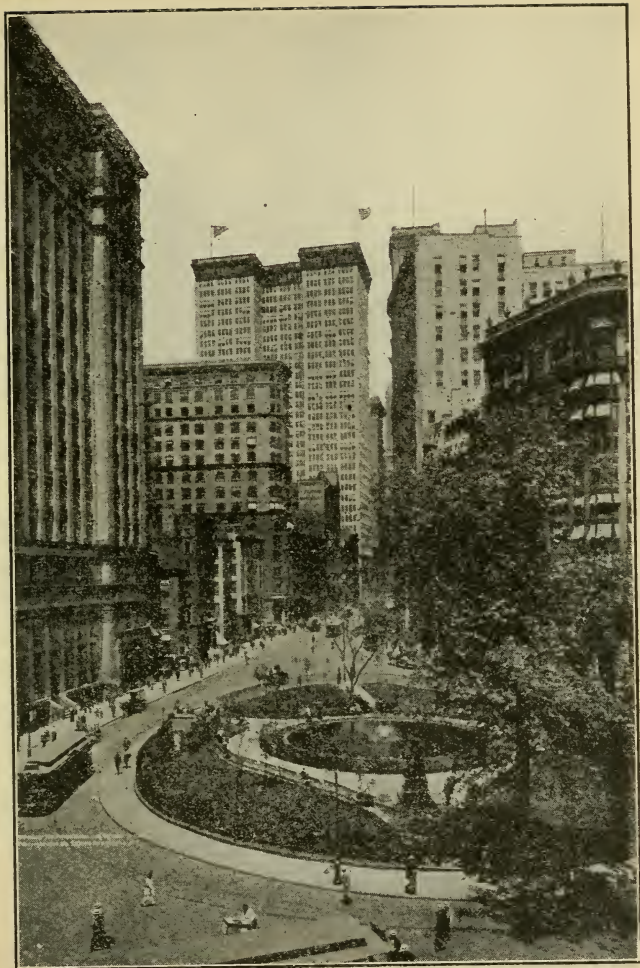
Bowling Green in front of the Custom House.
