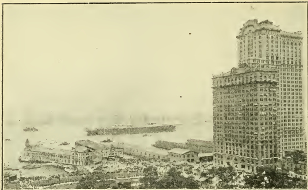
Battery Park. View of incoming liner. Whitehall Building on right
