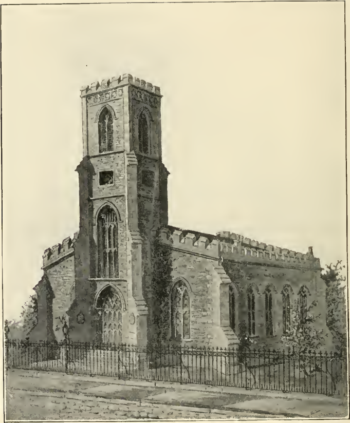
THE CHURCH OF THE STRANGERS, EXTERIOR.
