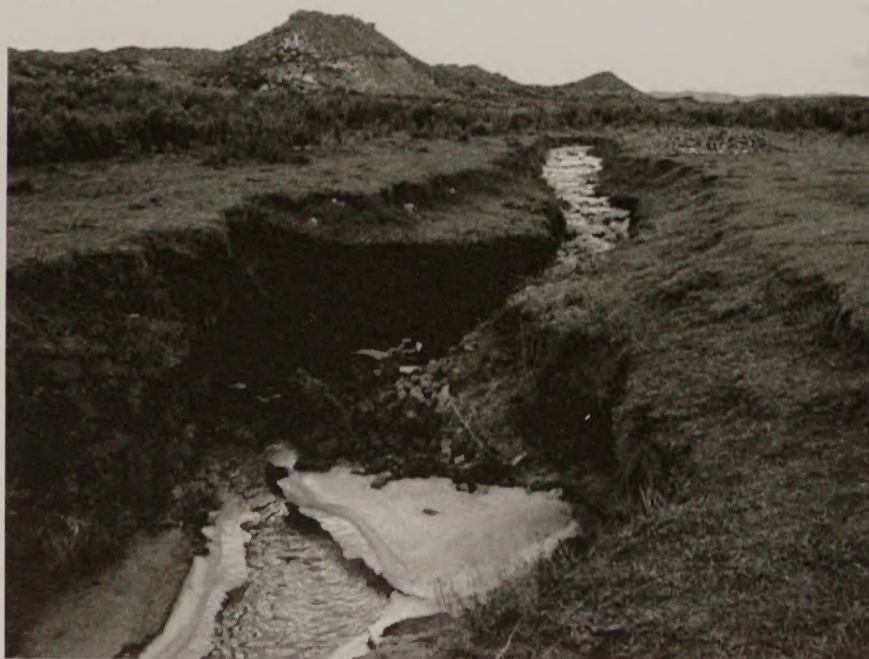
Figure 2: Riprap in Channel
