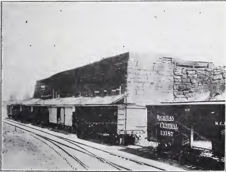
FIG. 6. 1 —Alvord and Company, Manlius, Onondaga County, New York. Old style of intermittent kiln now abandoned except in this district.
