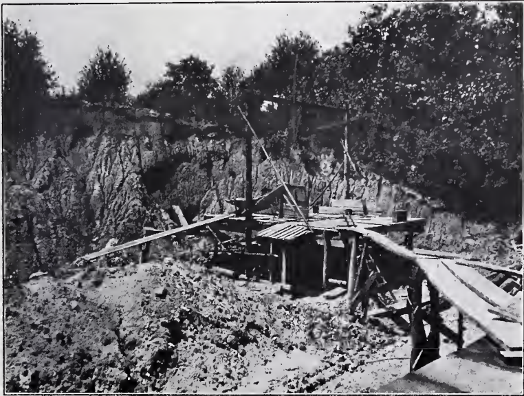
FIG. 12.—Shaft for mining refractory bond clay north of Anna, Ill.
