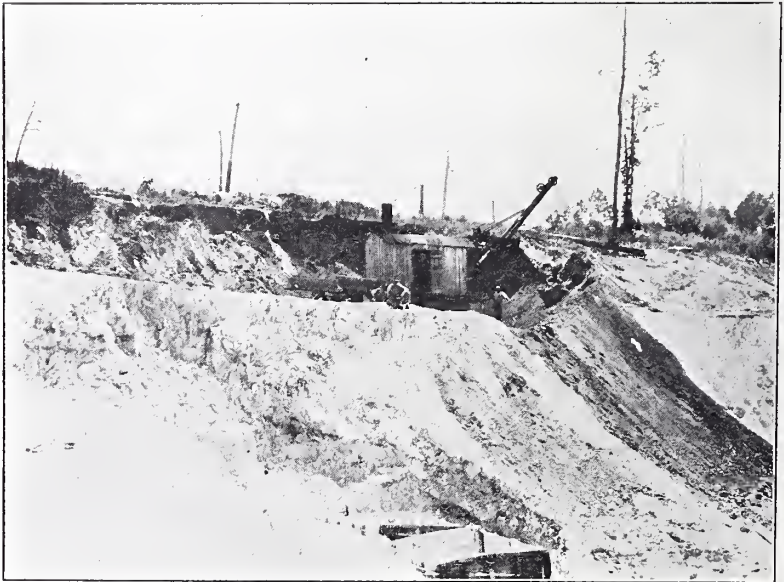
FIG. 1.—Removing sandy overburden from white clay with steam shovel at Gordon, Georgia.
