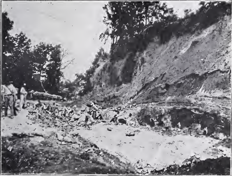
FIG. 8.—Digging ball clay near McKenzie, Tenn. Shows the heavy overburden that is removed.
