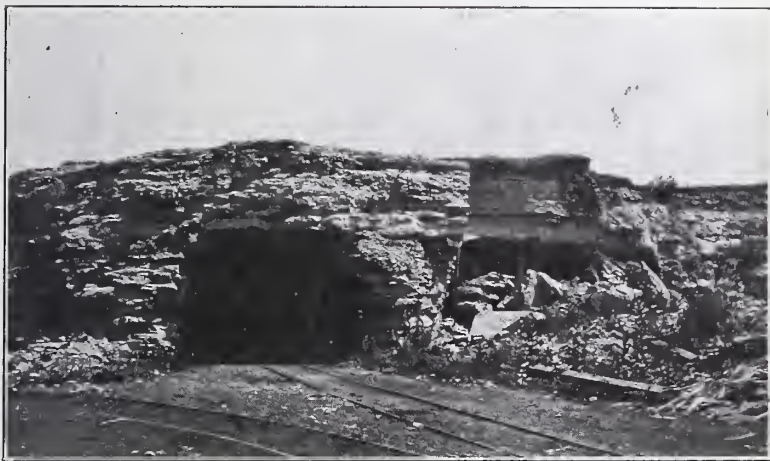
FIG. 3.—Opening in the cement layers at Akron, Erie County. A heavy layer of Onondaga limestone forms the roof.
