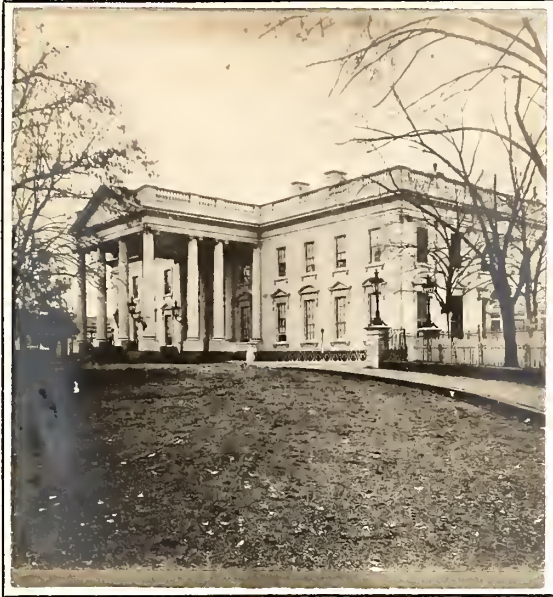
THE WHITE HOUSE During Lincoln's administration.
