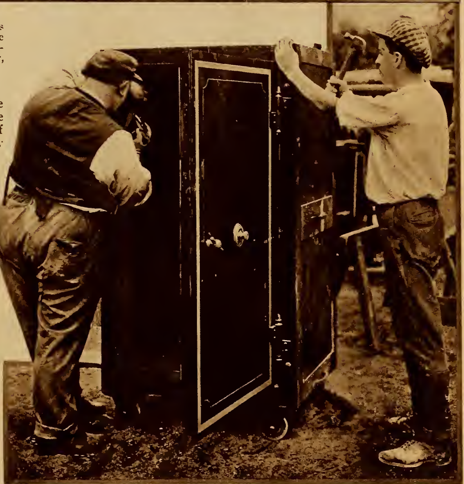
Building a safe to be blown up
