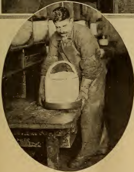
CRYSTALS OF PURE SILVER NITRATE. THE PORCELAIN BASKET CONTAINS ABOUT 1,000 OUNCES
