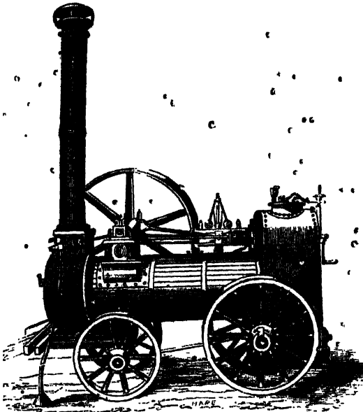
• Hornsby's Patent Six-horse Power Portable Steam-engine.
