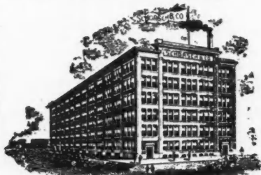
FACTORY 132 ND TO 133 RD ST & BROOK AVE
