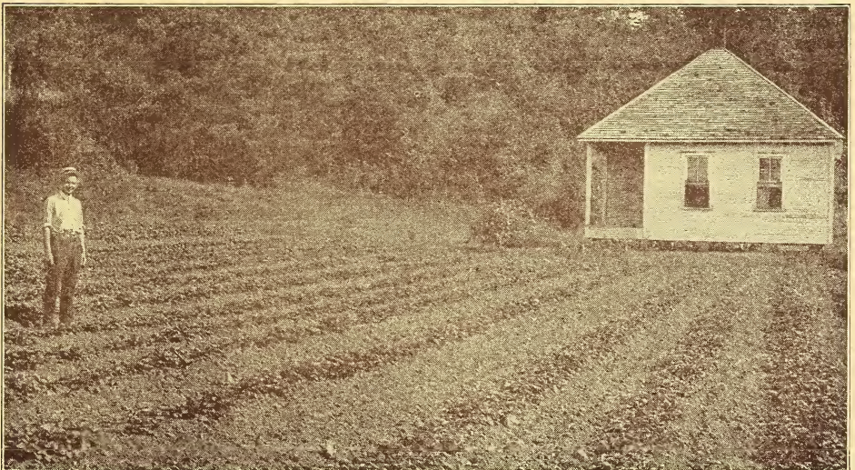
Manager Robert E. Blaylock, in corner of Breeding Bed. Note the growth of plants. (Picture taken in June.) Also note one of the smaller of ten tenant houses on plant farm in which we house our permanent and experienced help. Our employes live right in the strawberry fields, so to speak, ever ready to give our plant fields the care and attention to make them the world famous fruit producing plants they are.
