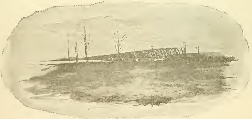
THE NEW STEEL BRIDGE ACROSS THE POTOMAC.
