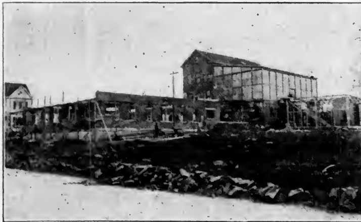
This photo shows the Solax plant in the process of expansion. The building in the background is the old plant, 150x150, three and one-half stories high. The studio accommodates five sets in a row. The present factory has an equipment sufficient to turn out one hundred thousand feet of positive film a week. The frame work to the right is an outdoor stage, used for light effects, and whenever work in the indoor studio reaches a state of congestion. The new two-story building in process of construction is on the left, also 50x100 and in it will be housed the factory and laboratory to be removed from the main building. The added facilities will make it possible to turn out about two hundred thousand feet of positive film a week. The space in the foreground, which is also the property of the Solax and Blanche companies, will be improved and fenced in by ornamented iron railings.
