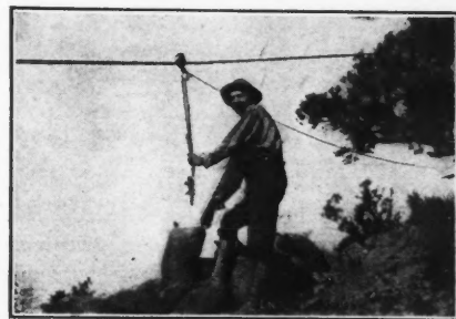
ATTACHING SLING TO SACK OF ORE ON IMPROVISED AERIAL TRAMWAY
