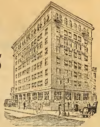
THE MAULE BUILDING
