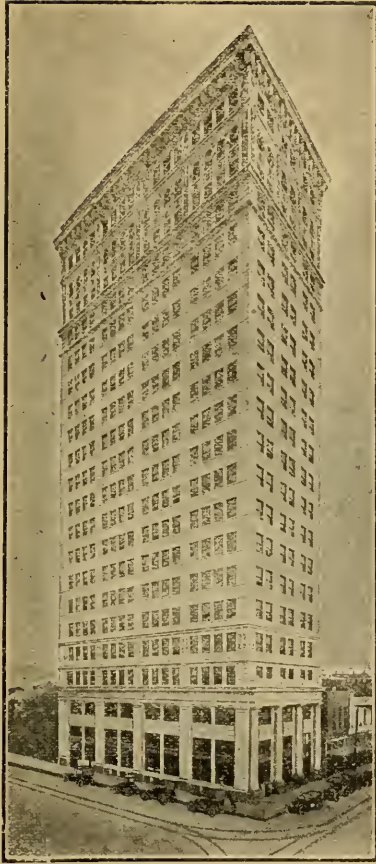
THE HOME OF THE AMICABLE LIFE INSURANCE CO. COMPLETED 1911
