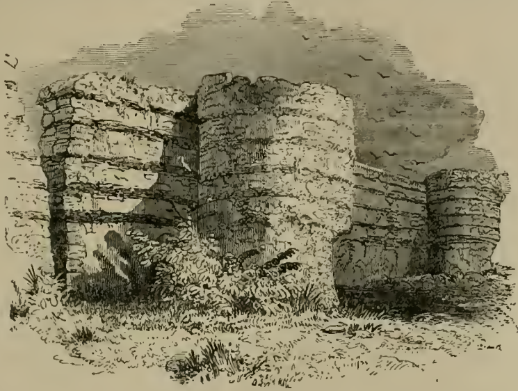
East Wall of Burgh Castle.
