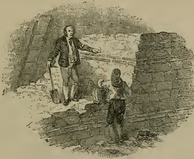
Part of the Roman Wall of London, excavated behind the Minories.
