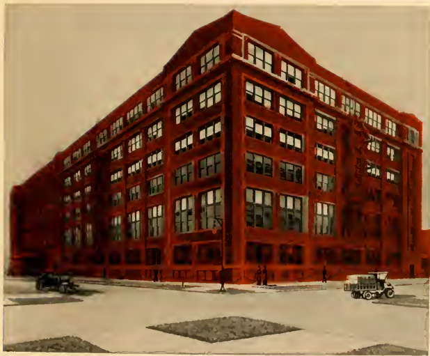
The Grocery Building, constructed of steel ribbed concrete. Seven acres of floor space
