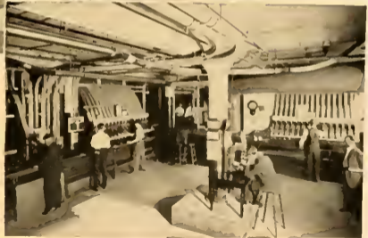
Station Pneumatic Tube System for transmitting orders and letters between all departments
