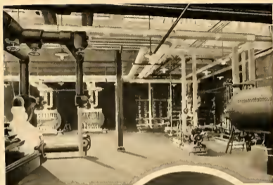
Water Cooling Plant
