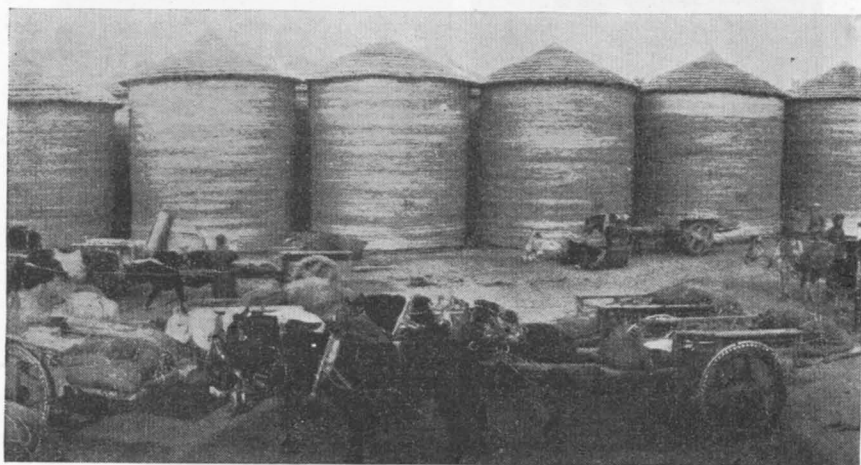
Figure 2.—Storage yard of a Chinese grain merchant near Kungchuling, Manchuria. More than 80 osier bins, each holding four carloads of soybeans, were in this yard.
