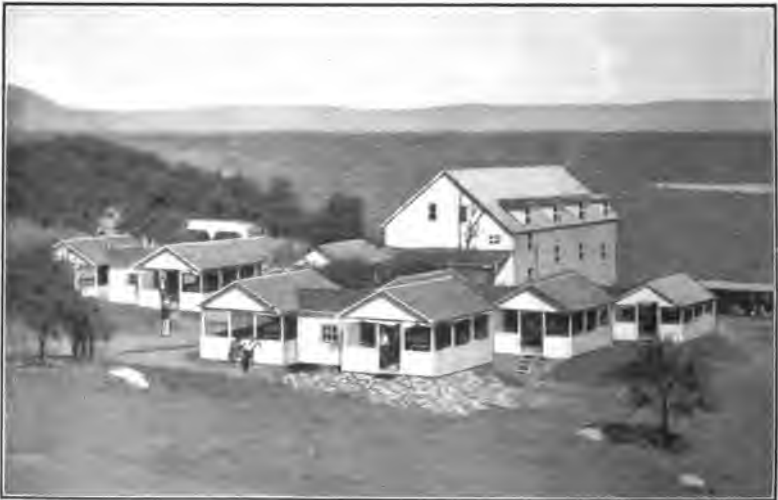
A sanitarium for tuberculosis. Notice the outdoor sleeping rooms.
