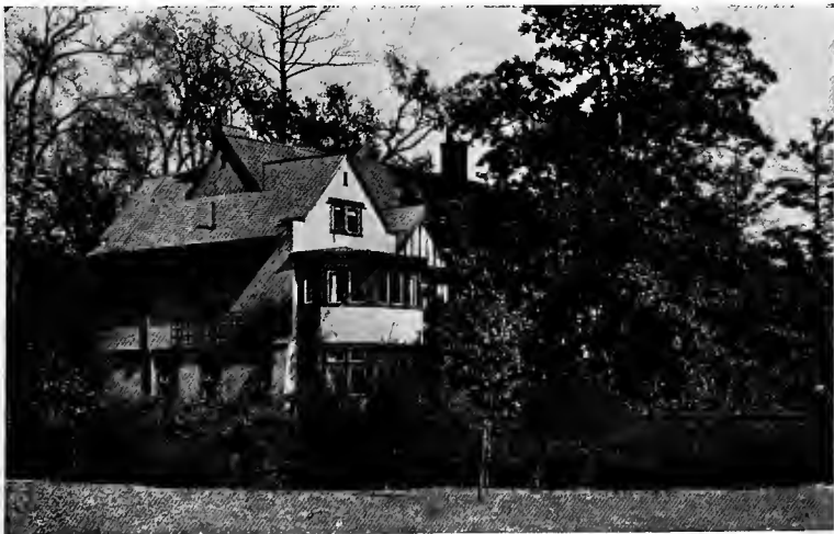
Half-timber work is best used as an accent for a gable or a bay here and there against plain plaster surfaces
