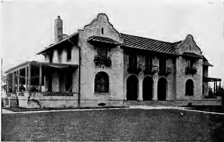
The arched doorways and gable ends are Mission characteristics; the porch is an addition made necessary by the lack of an interior court
