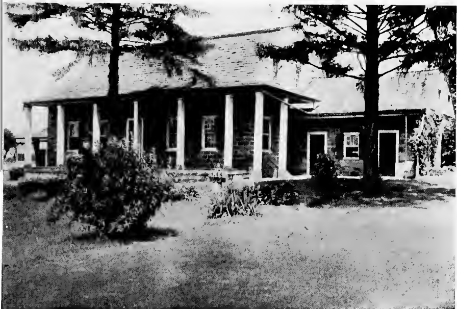
The Westervelt homestead, Cresskill, N. J., 1807. Where a piazza was introduced the overhang of the roof was extended and supported by slender wooden columns, square, octagonal or round
