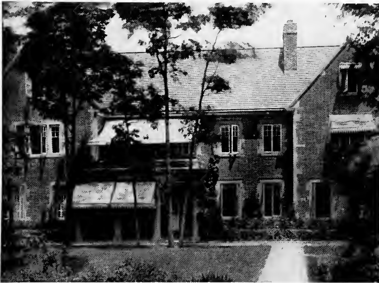
Mr. Chandler's house at Tuxedo, N. J. The Tudor brick house has about it an air of solidity and permanence that cannot be had with less enduring materials
