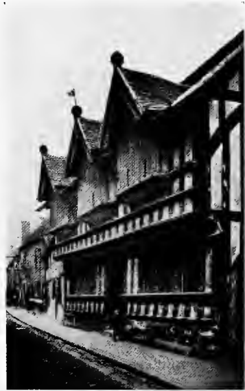
The overhang of the second story—a characteristic of the old work
