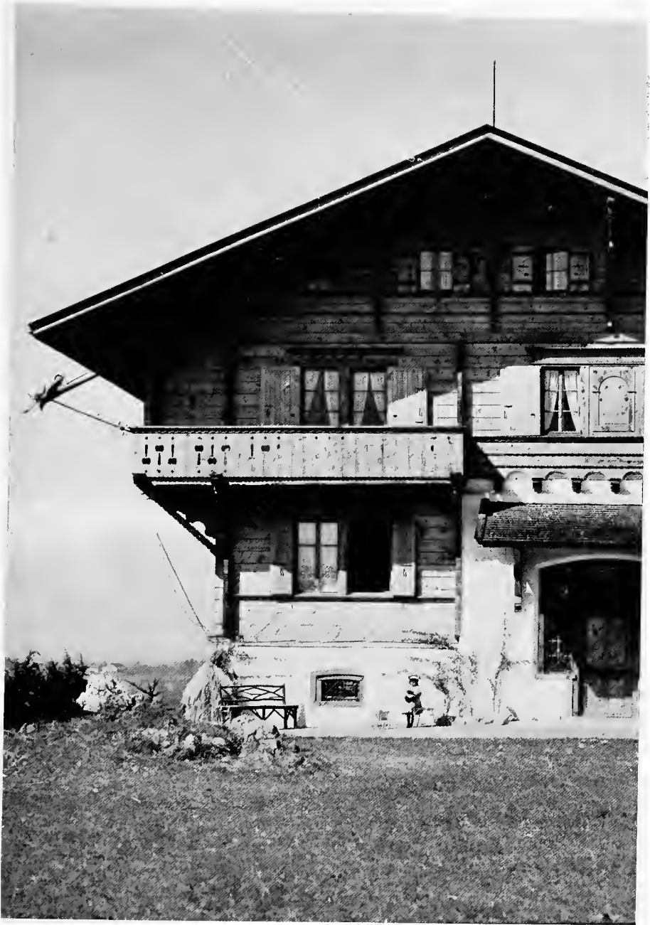
A modern Swiss chalet near Grisons which shows the recent use of stone and concrete in connection with wood
