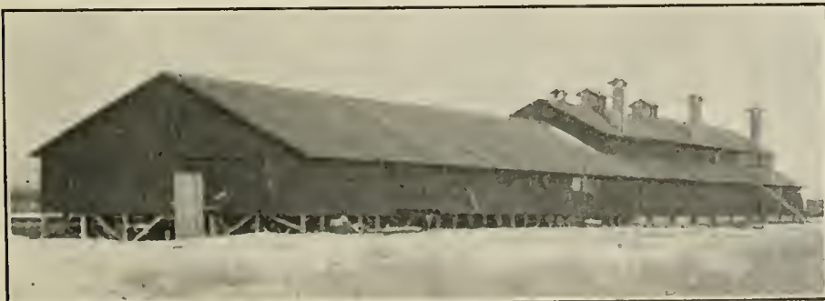
Large type of Northwest apple packing and air cooled storage house. Only the latter, however is frost proof
