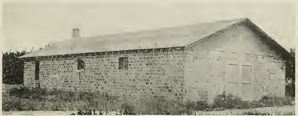
Small type of frost proof Northwest apple packing house. Although constructed of tile, this type of house is both poorly lighted and ventilated.
