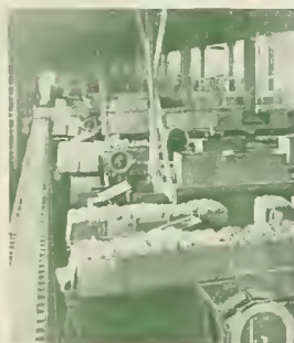
Portion of Standard System installed in the packing plant of the Peshastin Fruit Growers' Assn., Peshastin, Wash.
