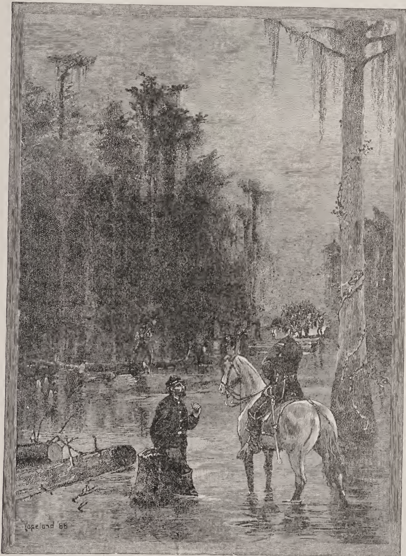
CONSTRUCTING A MILITARY ROAD THROUGH THE SWAMPS
