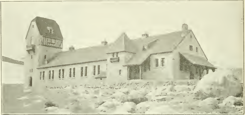
Fig. 32. Mt. Whitney Hatchery as it appears completed.
