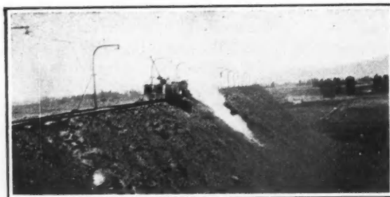
Midvale plant of the United States S. R. & M. Co. in Utah Electric locomotive hauling slag cars to dump
