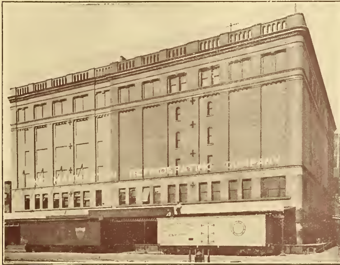
One of the Manhattan Cold Storage Warehouses.
